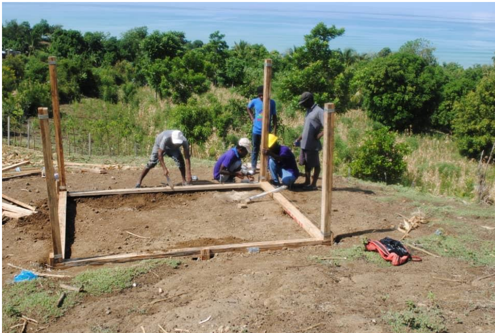
J635 goat shelter under construction at Les Anglais, Haiti (June 2020)
